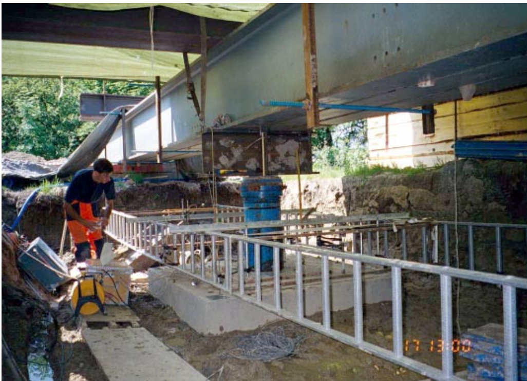
Fig. 83. Installation of the measuring system.
