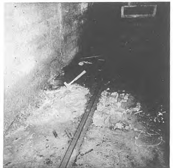
Figure 11. Heave of floor in a tunnel
