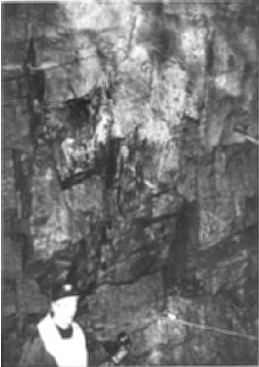
Fig. 10 Rätan tailrace tunnel, section 2000.
