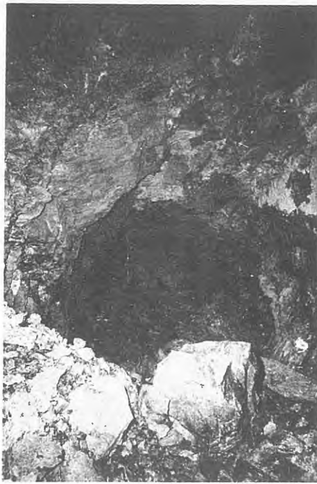
Figure 5. Example of a slide in a 6 \text{ m}^2 tunnel through a clay zone.
