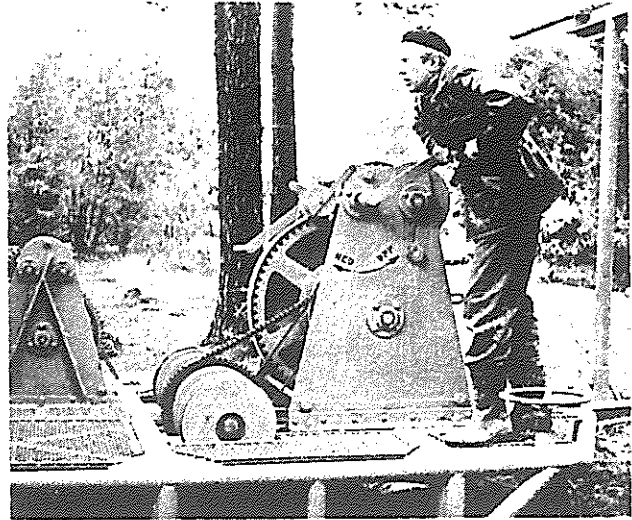
Fig. 3. Raising of mast
