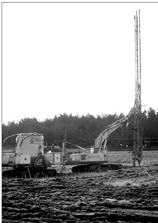
Figur 6. Pelarmaskin, LCM.
